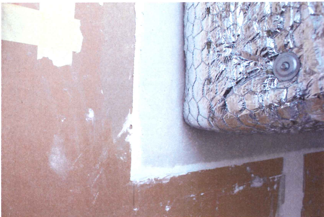
Photo 6: GPG sealant before testing.
