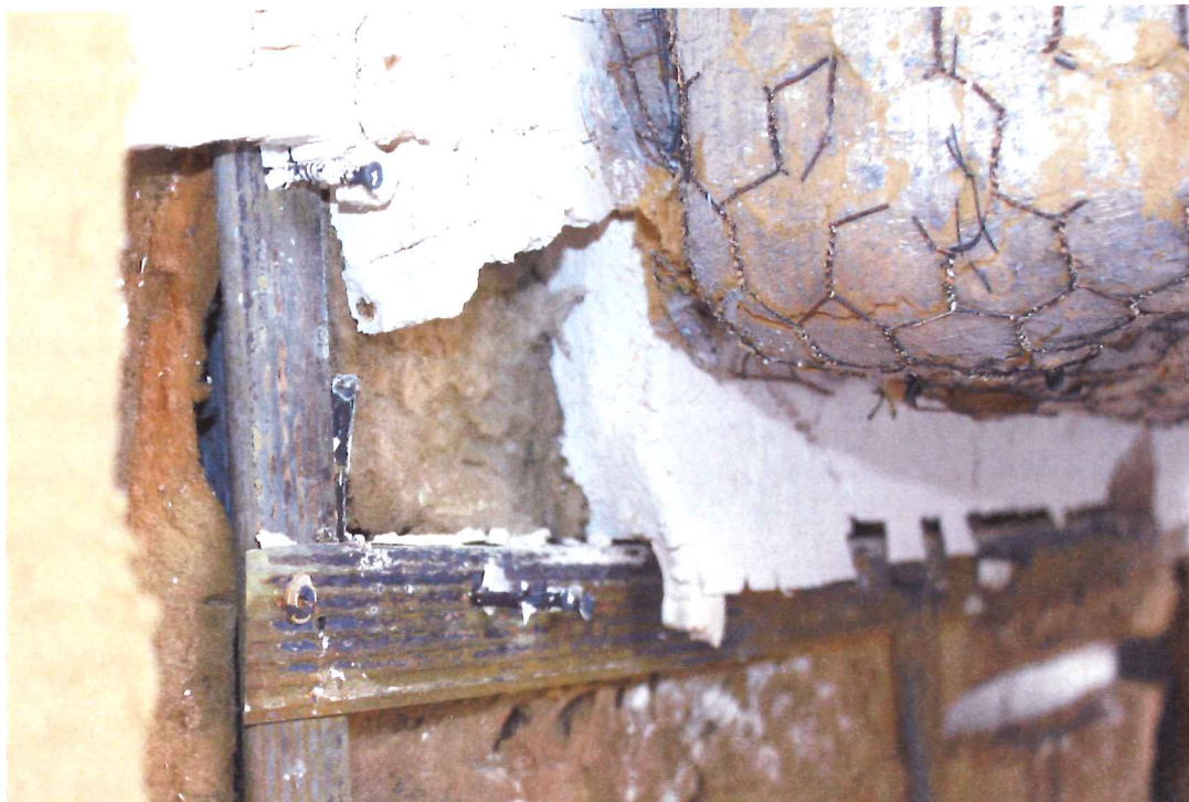
Photo 12: Exposed face one day after test. Note: detail of GPG sealant and stone wool in corner of duct B.
